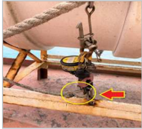
PORT & STBD life-raft painter was not connected to weak link. [Not properly stowed]
